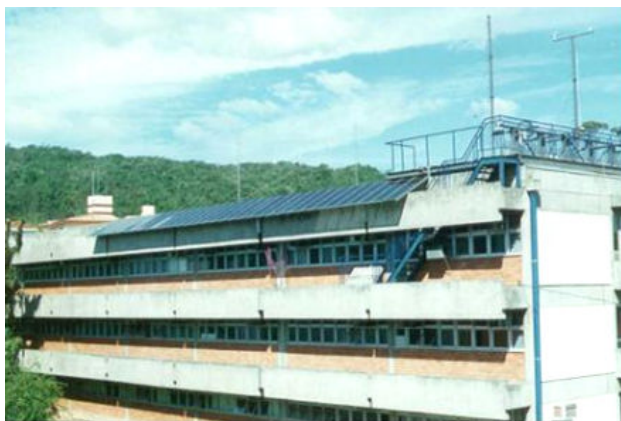
Figure 1 First grid-connected thin film BIPV system installed in Brazil (1997), with a mix of 54 opaque and 13 semitransparent, double-junction, same band gap, unframed amorphous silicon (a-Si) PV glass-glass modules.
